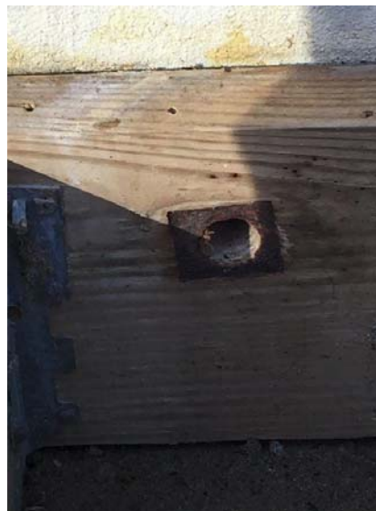
eLOMC – Photos of deck supports disconnected from residence
