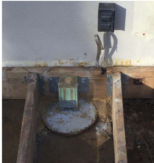
eLOMC – Photos of deck supports disconnected from residence
