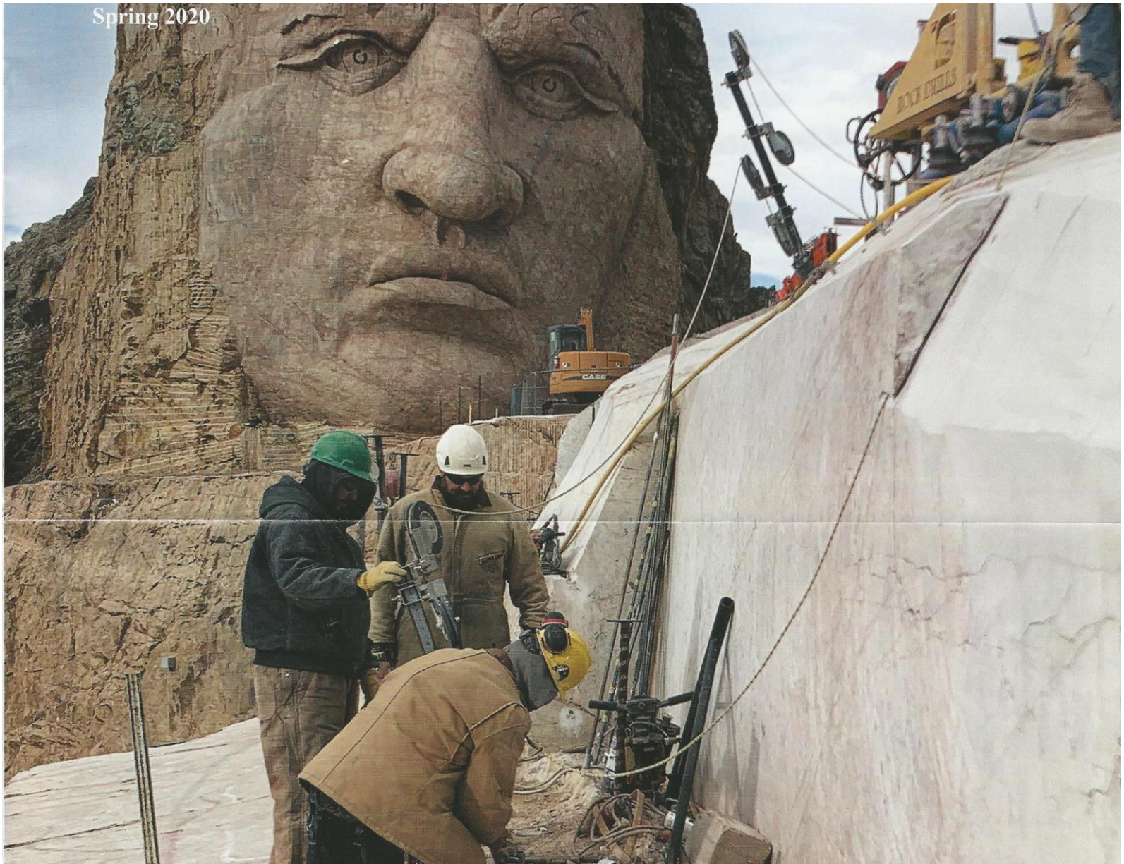
Using diamond wire saws Progress, Spring 2020
