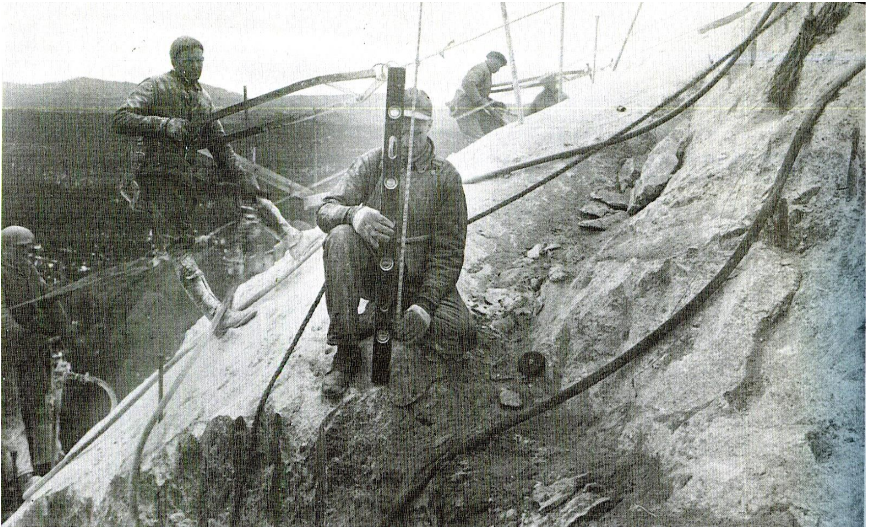
Pointer transferring measurements to Washington's head, fall 1927. (Smith, The Carving of Mount Rushmore , p. 162)
